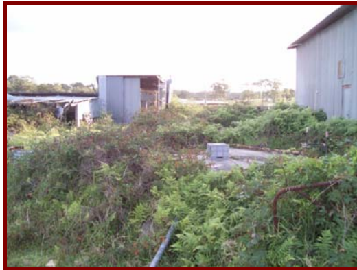
Photo 3 – Former chicken shed and filling
